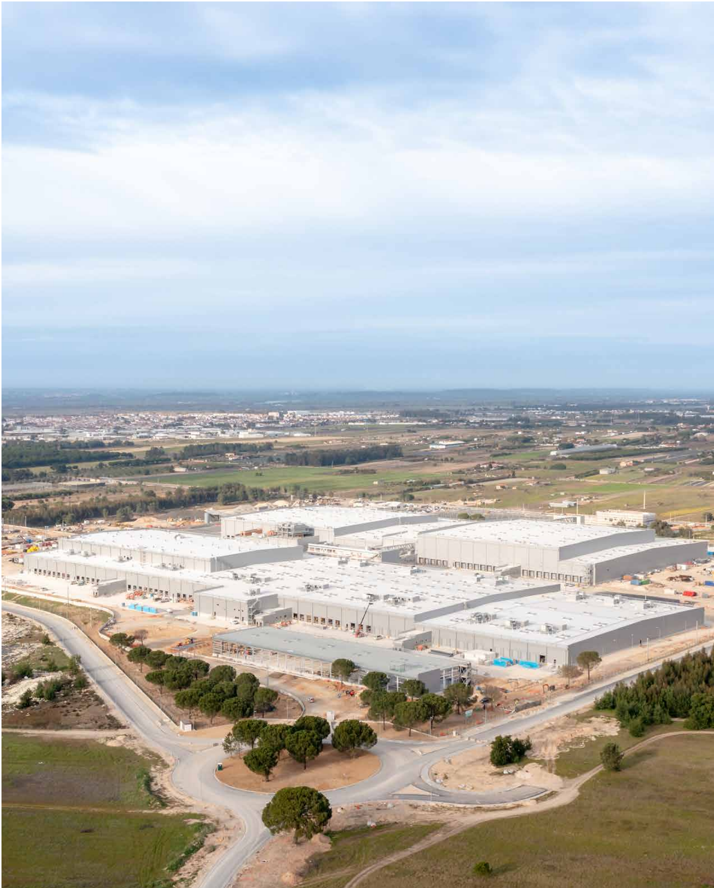
Aerial view of the logistics centre in Almeirim, Santarém, currently under construction.
