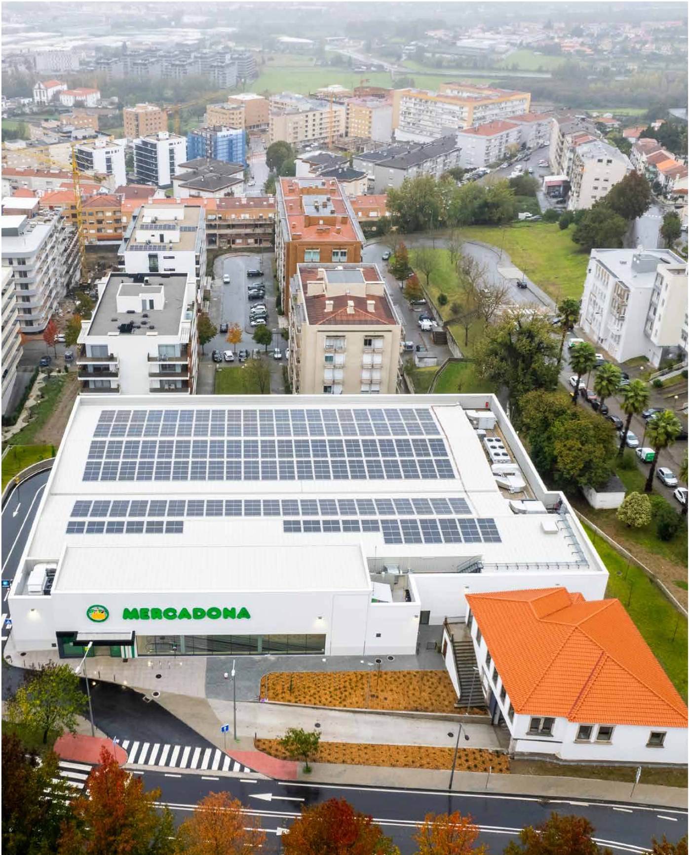
Aerial view of the Quinta de Santa Bárbara supermarket in Braga, adjacent to a restored traditional Minho house. In addition, a barn was restored and relocated to the Braga Pedagogical Farm.
